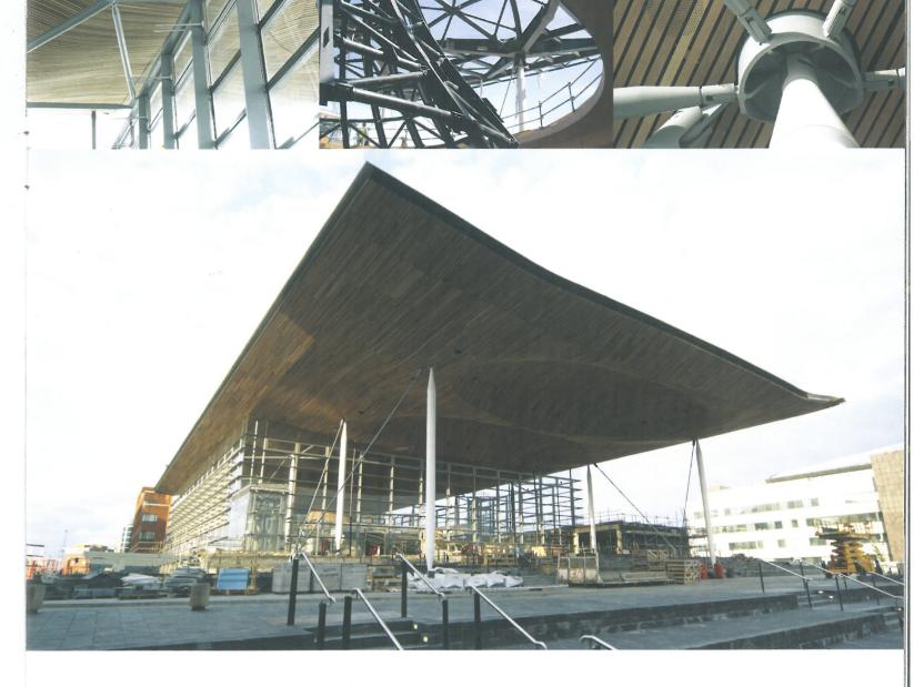
sections for transport and then to combine these on site at ground level into the heaviest assemblies suitable for craneage, keeping lifts to a minimum.
