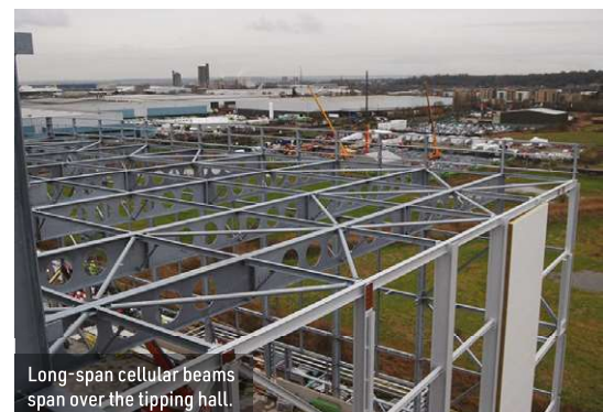
Another crane beam is supported by a series of lattice columns.
