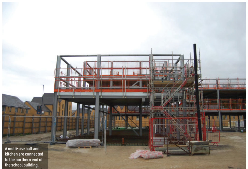
Steel beams support a precast flooring solution throughout the school.
