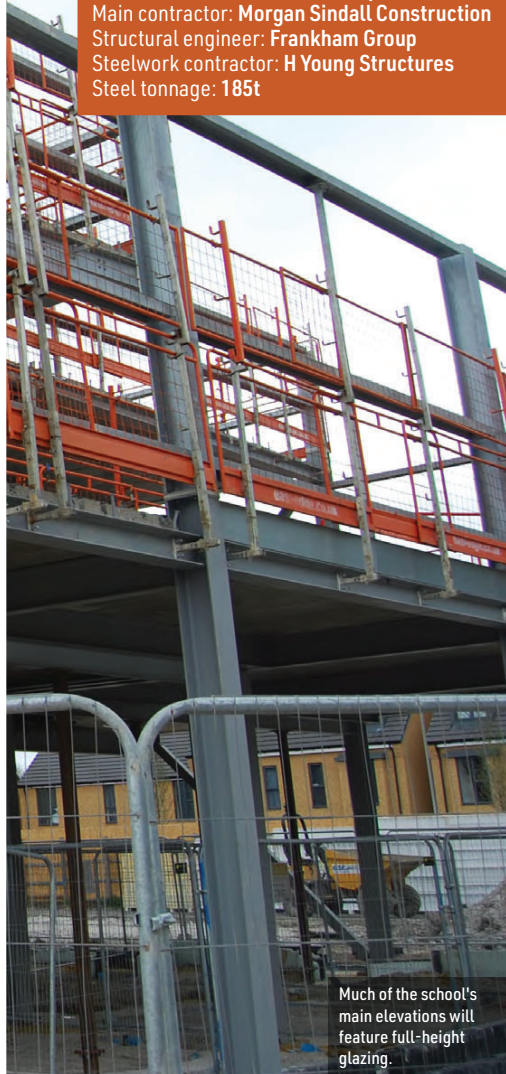
With the ground works completed, the steel frame erection begins.
