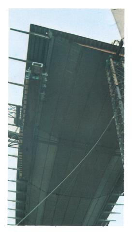
proximately at 2ft centres which are supported by full depth diaphragms, generally at 14ft centres. The roadway and cycle tracks are surfaced with 1½in mastic asphalt. The footways consist of steel panels surfaced with ½in mastic asphalt.
