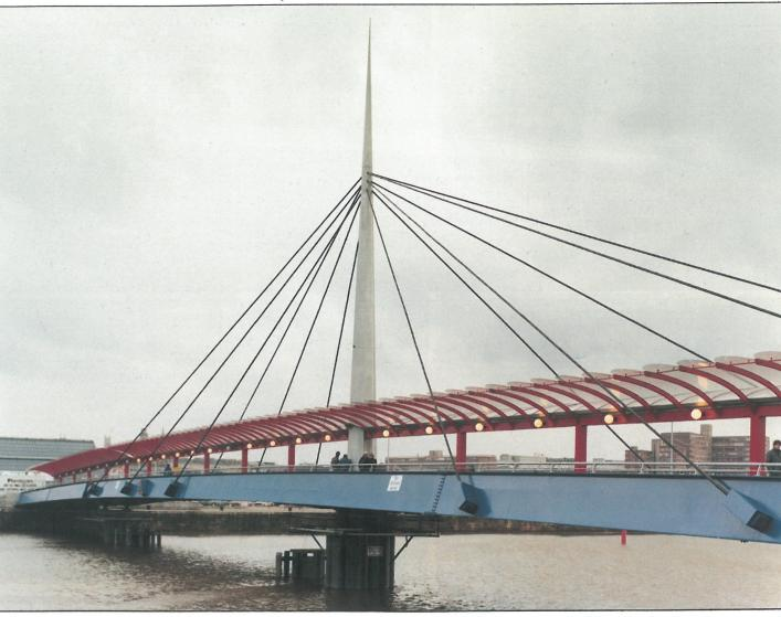
With the aid of wire ropes and sliding sheaves one cylinder pulls the bridge round while the other restrains it. The operation is controlled from a small consol mounted in the side of the pylon and from the start of releasing the locking dowels the time for opening is less than five minutes. The required overall response time for the bridge to be open for navigation is 15 minutes. To close the bridge the sequence is reversed.
