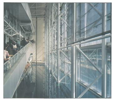
structure was stabilised longitudinally in the central bay of the envelope by crossbracing in the walls and across the roof.
