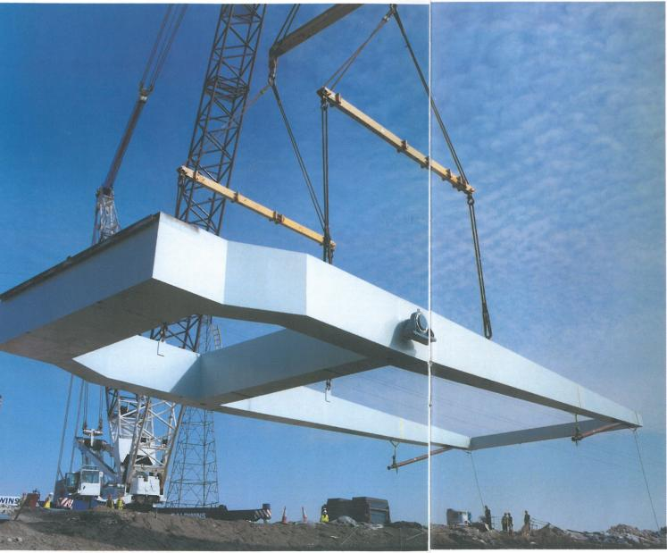
measuring 13m wide by 33m long by 3.5m high, were assembled on the temporary overburden within working radius of the main erection crane. The counterarms (140 tonnes each) were constructed on the lower approach road and transported to the crane using multi-wheeled transporters.
