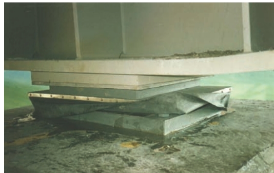
Figure 3 Guided bearing (with skirt)
