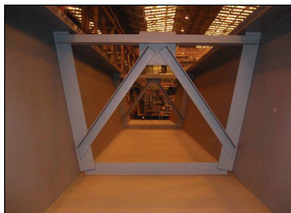
Figure 2 Internal view of a steel box girder where longitudinal stiffeners were avoided by the use of thicker plates
