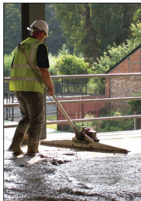
Concrete surface floated smooth
