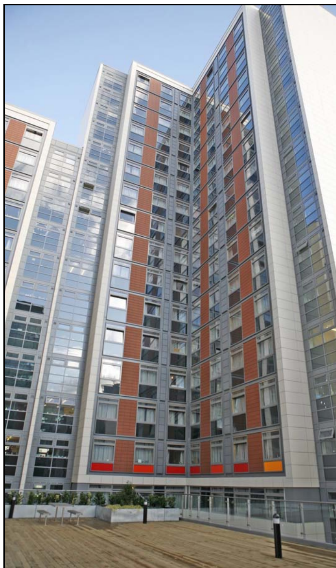
Seventeen storey modular building at Paragon project
