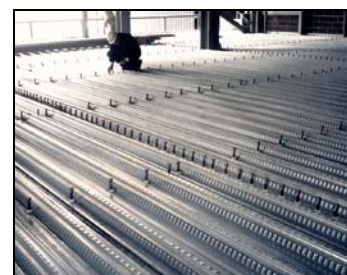
Composite deck on steel beams
