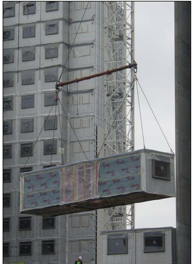
Lifting an open-sided module
