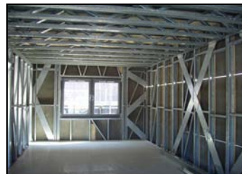
Light steel framing system
