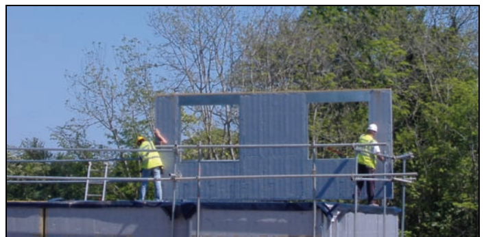
Erection of wall panel
