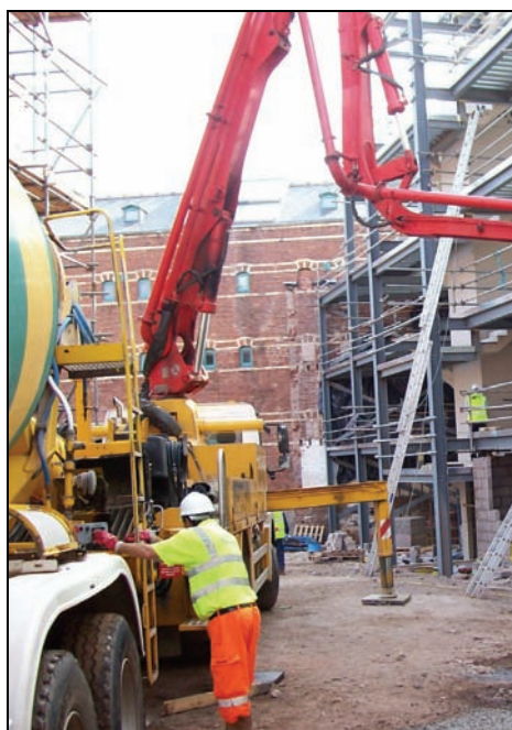
Concrete pumped onto decking
