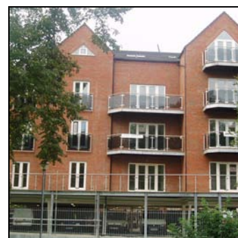
Car park below apartments
