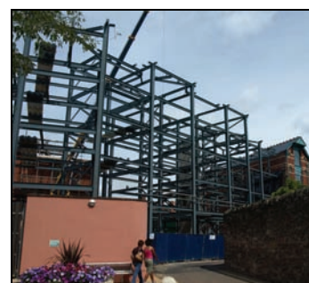
Structural steel frame
