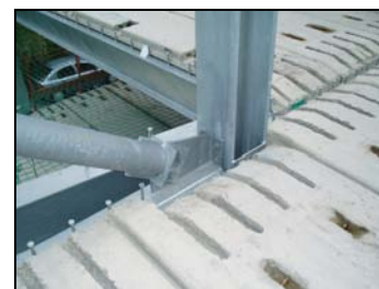
Hollow core units on steel frame
