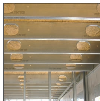
Light steel joist
