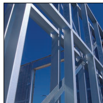
Light steel framing
