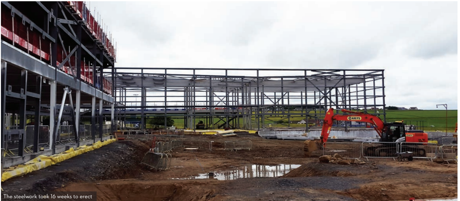
The steelwork took 16 weeks to erect
