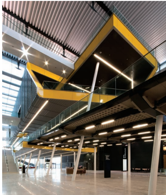
Conference areas are situated in a raised box accessed directly from the main circulation area.
