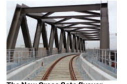
The New Cross Gate flyover.
