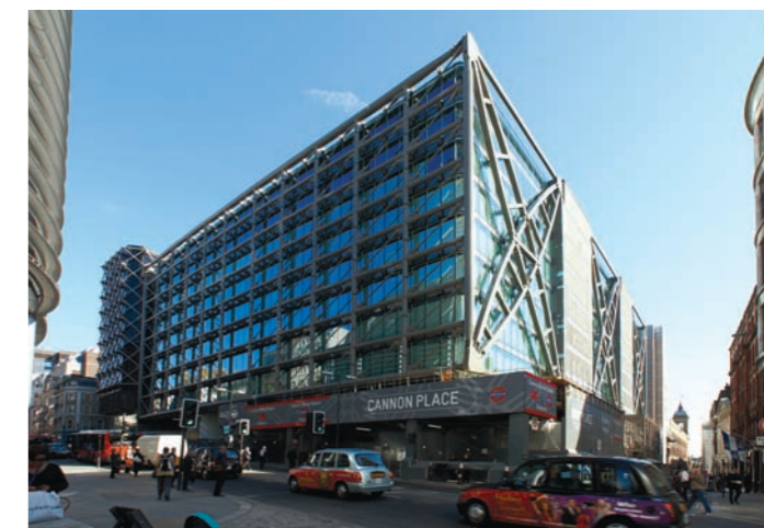
The steel structure is fully expressed, with curtain walling inside the structural frame.
