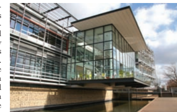
The steelwork frame has been designed to accept an additional three levels of mezzanine to allow future expansion by M&S.
