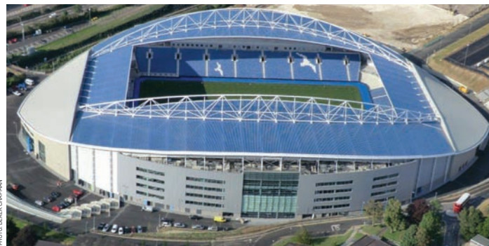
The east and west roofs are supported by 170m-long arched and leaning roof trusses.
