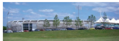
The rear elevation has a timber louvred facade.
