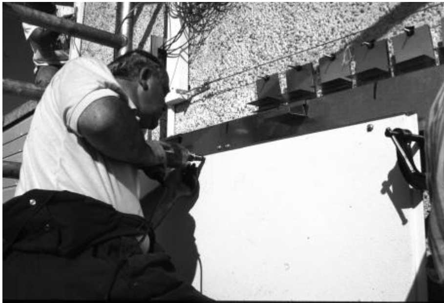
Figure 3.5 Galvanized steel coupons installed behind the over-cladding panel
