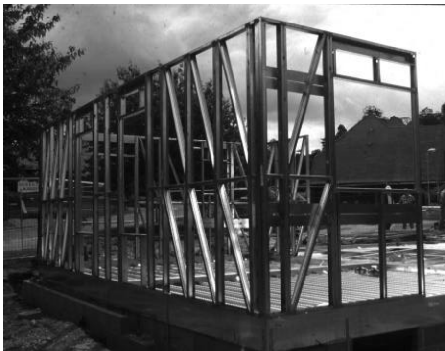
Figure 1.1 Light steel framing in housing
