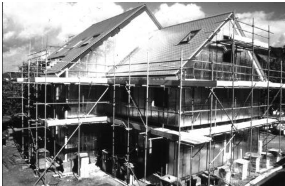
Figure 1.2 Warm frame construction showing external insulation
