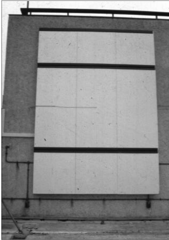
Figure 3.4 Over-cladding panel at Edinburgh University
