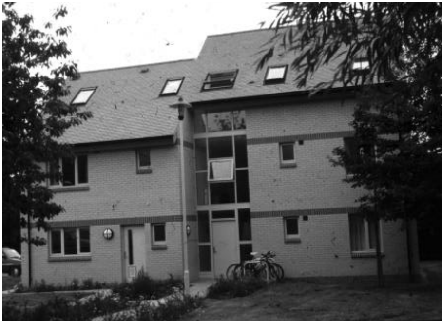
Figure 3.6 Oxford Brookes Demonstration Building
