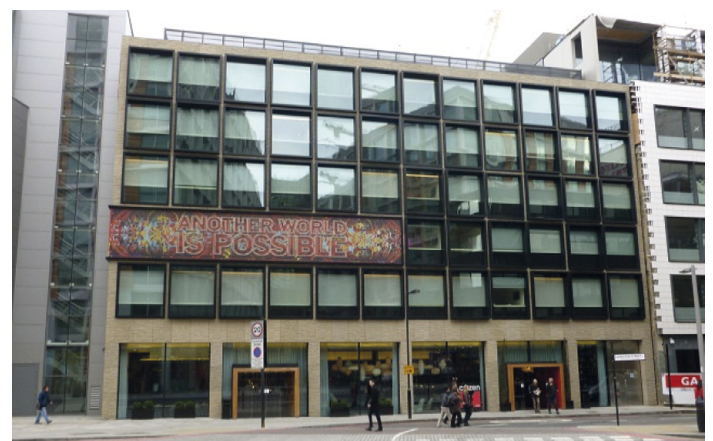
Figure 4: Completed modular hotel on Lavington Street, Southwark showing the use of a first floor steel podium structure
