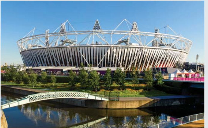
Some 2,500 of the 3,850 tonnes of steel tubing in the Olympic stadium's roof trusses was reclaimed from old gas pipes.
