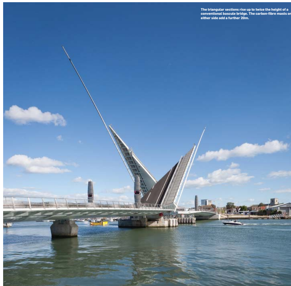
The 2.4m-wide walkways on either side of the bridge are separated from traffic by a stainless-steel screen that is designed in a wave form.
