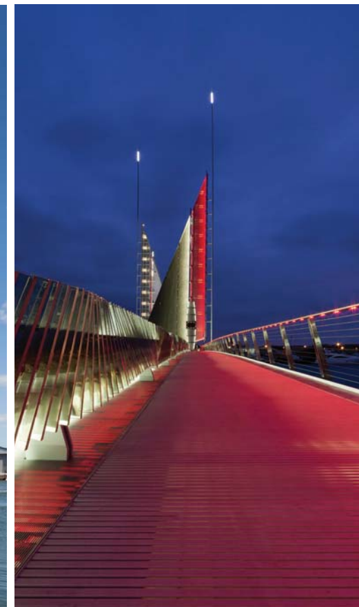
The 2.4m-wide walkways on either side of the bridge are separated from traffic by a stainless-steel screen that is designed in a wave form.
