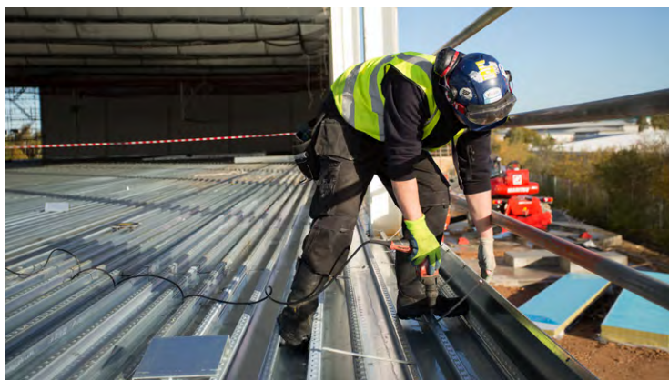
Figure 4.16 Setting out of edge trim
