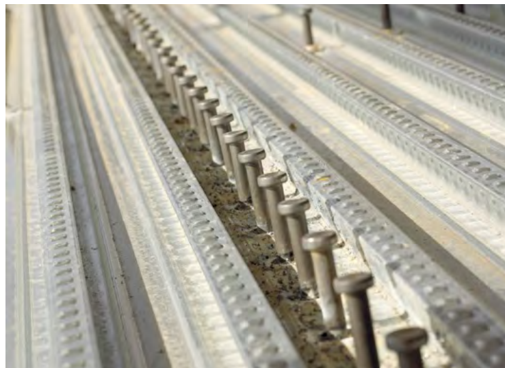
Figure 5.8 A run of stud shear connectors
