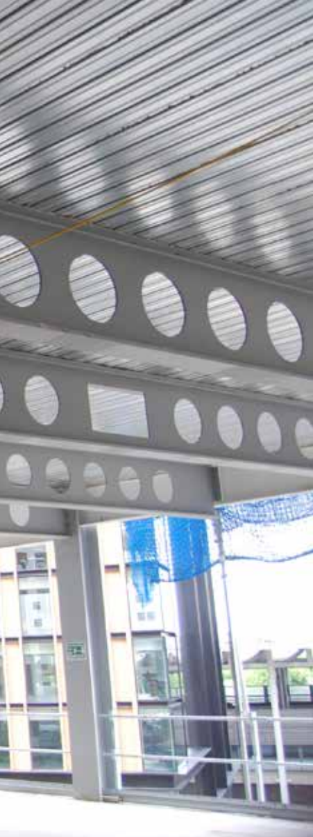
Steel's long span qualities are utilised in distribution warehouses
