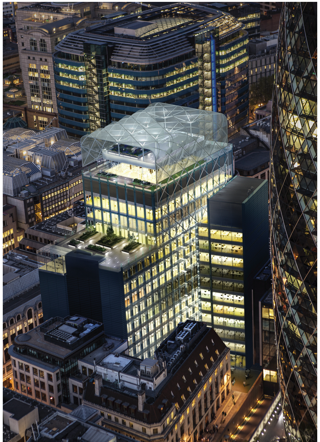
Right 6 Bevis Marks is topped with a spectacular canopy over a sky garden with views over the City of London and beyond.
