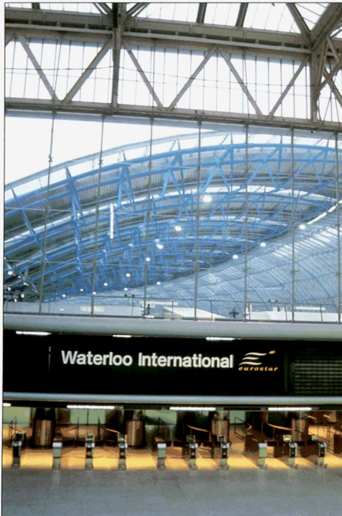
Waterloo International Terminal
