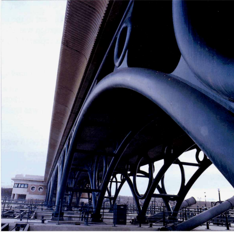
Circular infill casting
