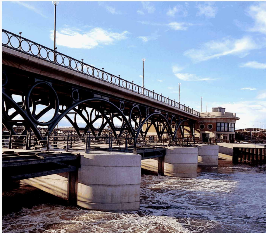
Tees Barrage Bridge
