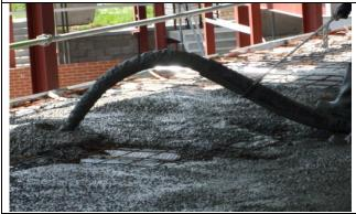
The outlet pipe should be moved frequently and carefully so that concrete heaping is minimized. A minimum of 2 people are required for this operation, one to hold and manoeuvre the outlet pipe, the other to shovel away excess concrete. No more than 4 workmen should be present around the pipe outlet during pumping!
