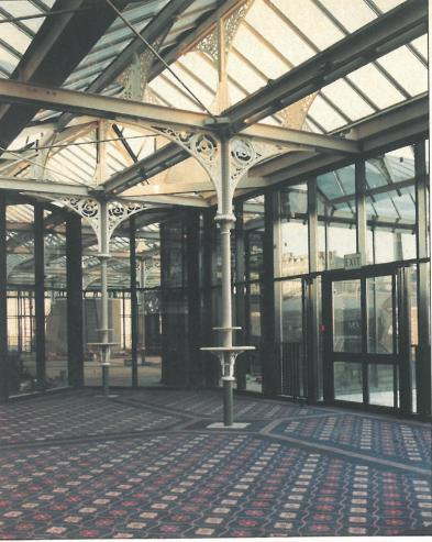
means of lateral stability within the foyer area, and the requirement for clean and well-aligned connection details for the RHS raf-ters and purlins, in view of the visual prominence of the structure. In order to comply with these requirements, a horizontal diap-hragm was formed at column head height. The forces on the foyer
