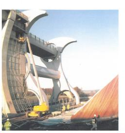
By any measure the Falkirk Wheel is an unusual structure. Weighing approximately 1400t without water it is a large machine. Raising and lowering boats in a rotary motion makes it unique.
