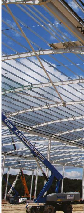
Making sure the steel frame was erected efficiently has a knock-on effect to the rest of the scheme. As once the steelwork is up, or partially up, the follow-on trades, such as cladding and roofing, are able to begin their work.
