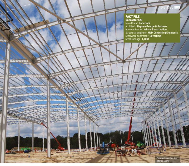
up 3t each, the rafters are typically 838mm x 292mm 226mm UBs, weighing 4.3t when spliced together.
