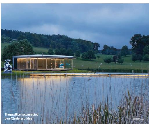
filled structural members and a patented integrated roof and rear wall stainless steel cladding system. The structure is formed from three-pin portal frames at 3m centres, made from bespoke stainless steel sections for the rear and top elements. This allows the front members to be much slimmer pinended stainless steel Circular Hollow Section (CHS) columns, minimising their visual impact on the fully glazed façade.
