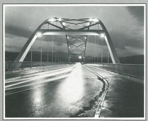
This new bridge is the third to cross the Kyle of Sutherland. The first was built in 1812 but was swept away by floods in 1891; the second was opened in 1892 but increased loads combined with the effects of corrosion and scour led to the decision to build a new bridge. The specification called for a 7.3m carriageway with a 2m footpath each side, full HB loading and resistance to winds up to 140 mph
