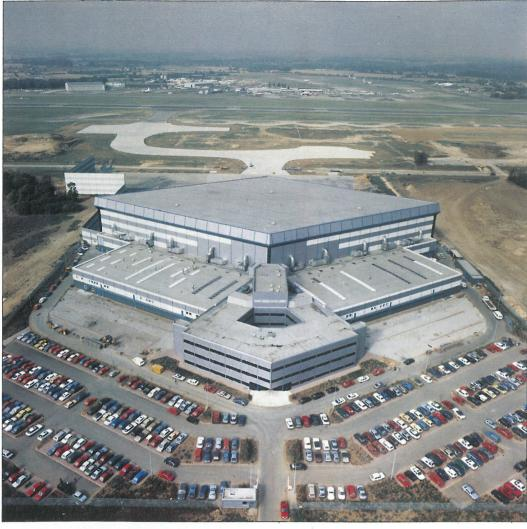
There are two basic geometric requirements for the main hangar building. Firstly, it was to be capable of housing for maintenance purposes, two Boeing 747 400 series aircraft under a single span roof without internal columns. Secondly, it was to impose the minimum possible visual intrusion on the Essex skyline.
