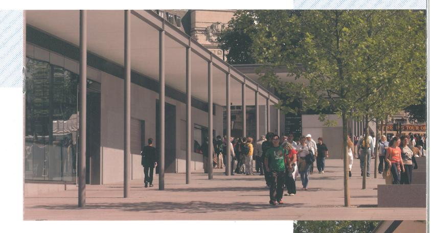
Stability for all three structures is generally achieved by vertically cantilevering columns in conjunction with cross-braced roofs.
