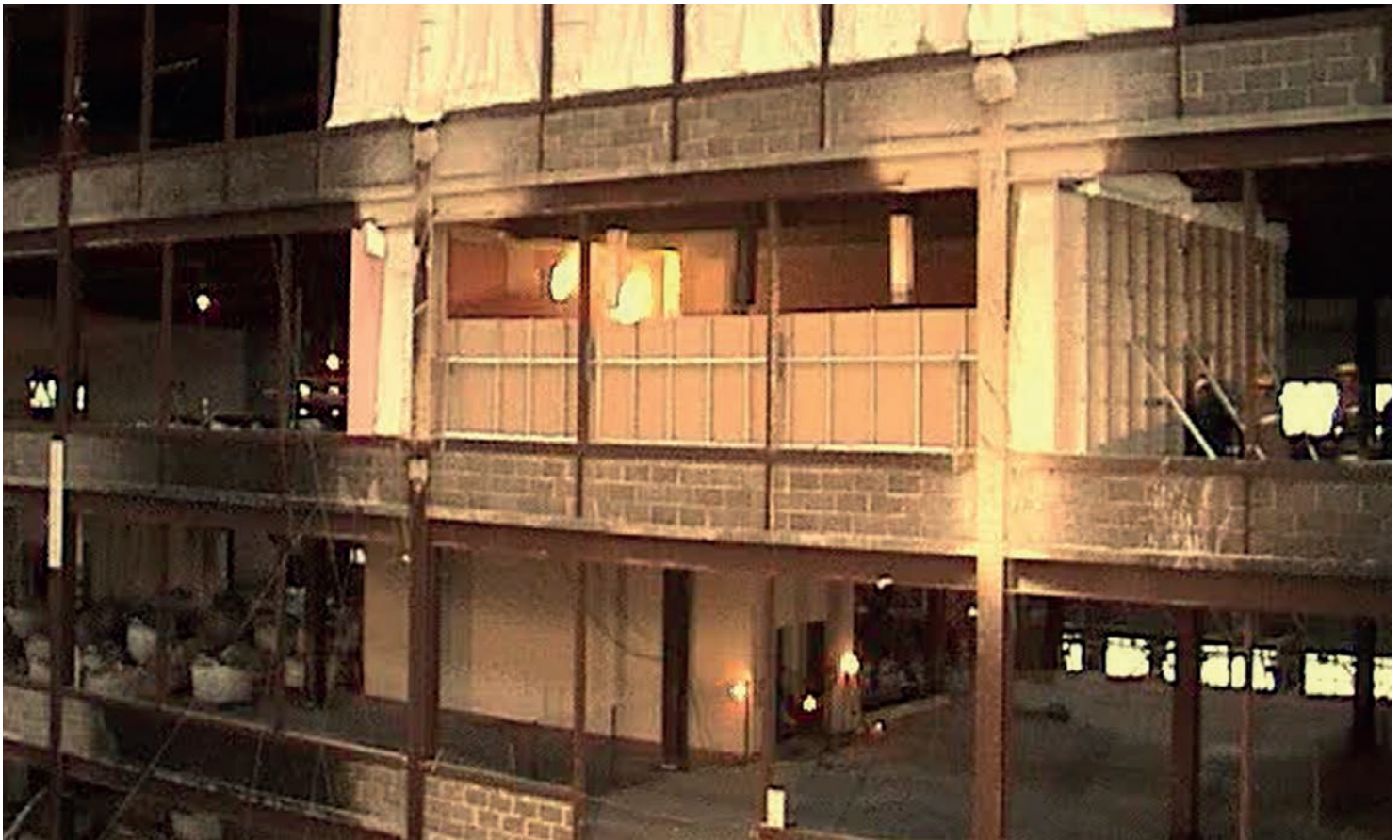
Fire tests carried out by the BRE at Cardington in the 1990s supported the finding that interactions between structural members increase the overall level of fire resistance
