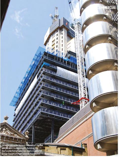
through these raking columns and to stop the frame from splaying outwards, there are large complex connections and embedment plates cast in to the concrete core to resist the tension generated in the sixth-floor steelwork and compression in the first-floor steelwork," explains Robert Bird Group Project Director Matt Quilty.
