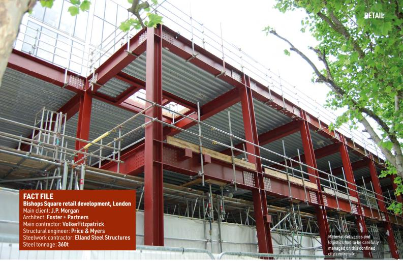
basement wall. However, the main elevation containing the shopfronts has no existing columns or wall beneath the new steel frame's perimeter line and so a series of trusses has been installed along this façade.
